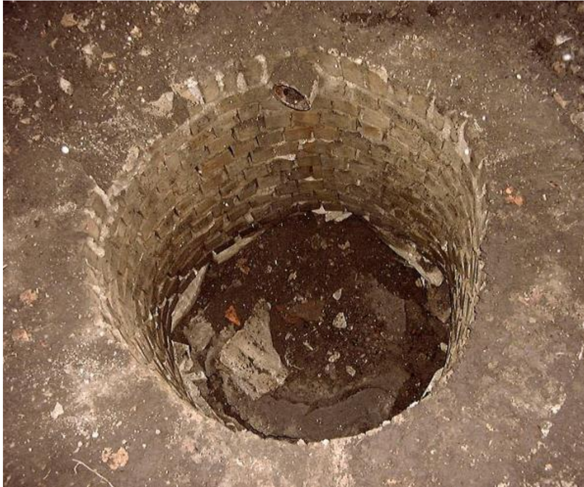
Dry well for stormwater infiltration
